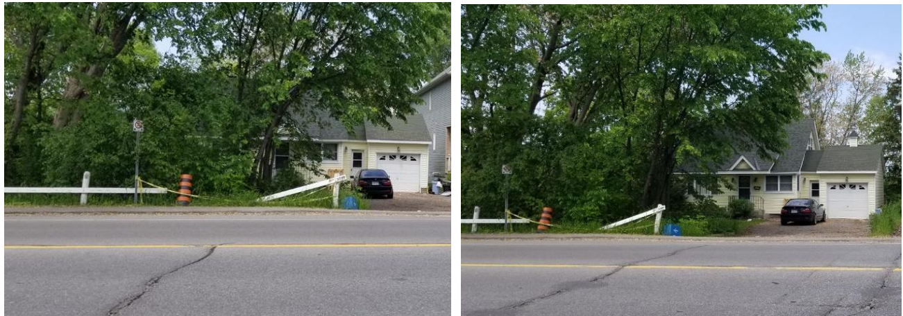
Figure 2-2 Existing detached dwelling, looking north from Richmond Road
