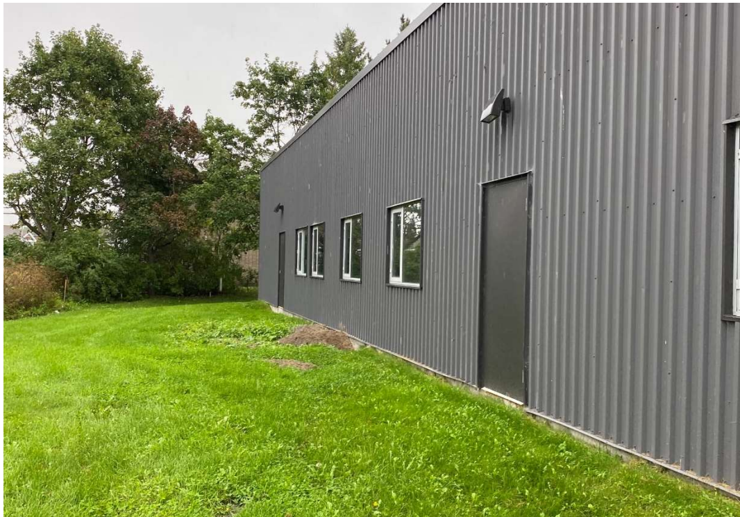
Photograph 2: View of Phase I Property looking east
