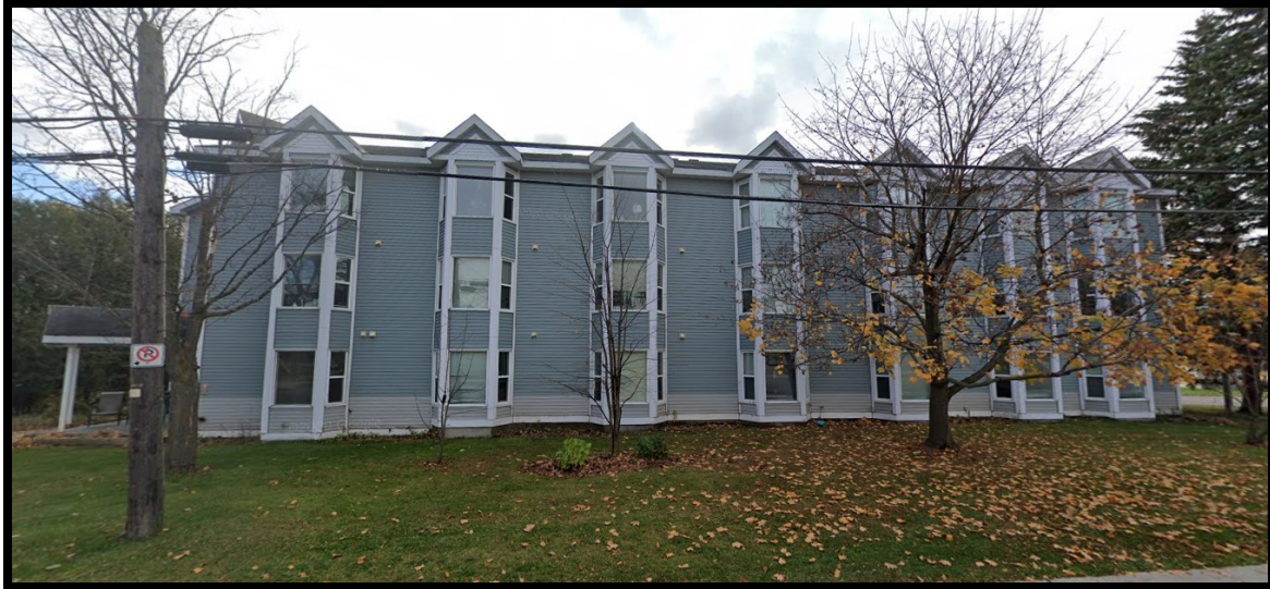
Fig. 2. Blackburn Seniors Residence Ottawa located north of the subject property.
