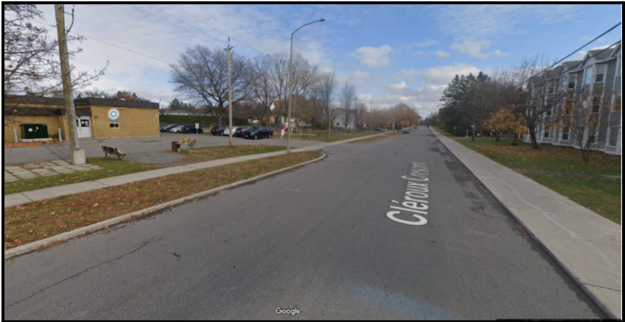
Property at the Cleroux cres / Innes rd.
