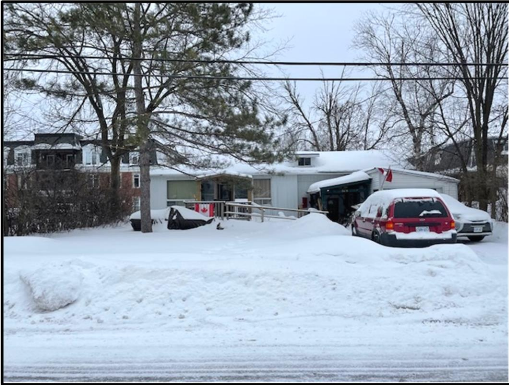
Photograph 1: The subject building at 2458 Cleroux, looking south.
