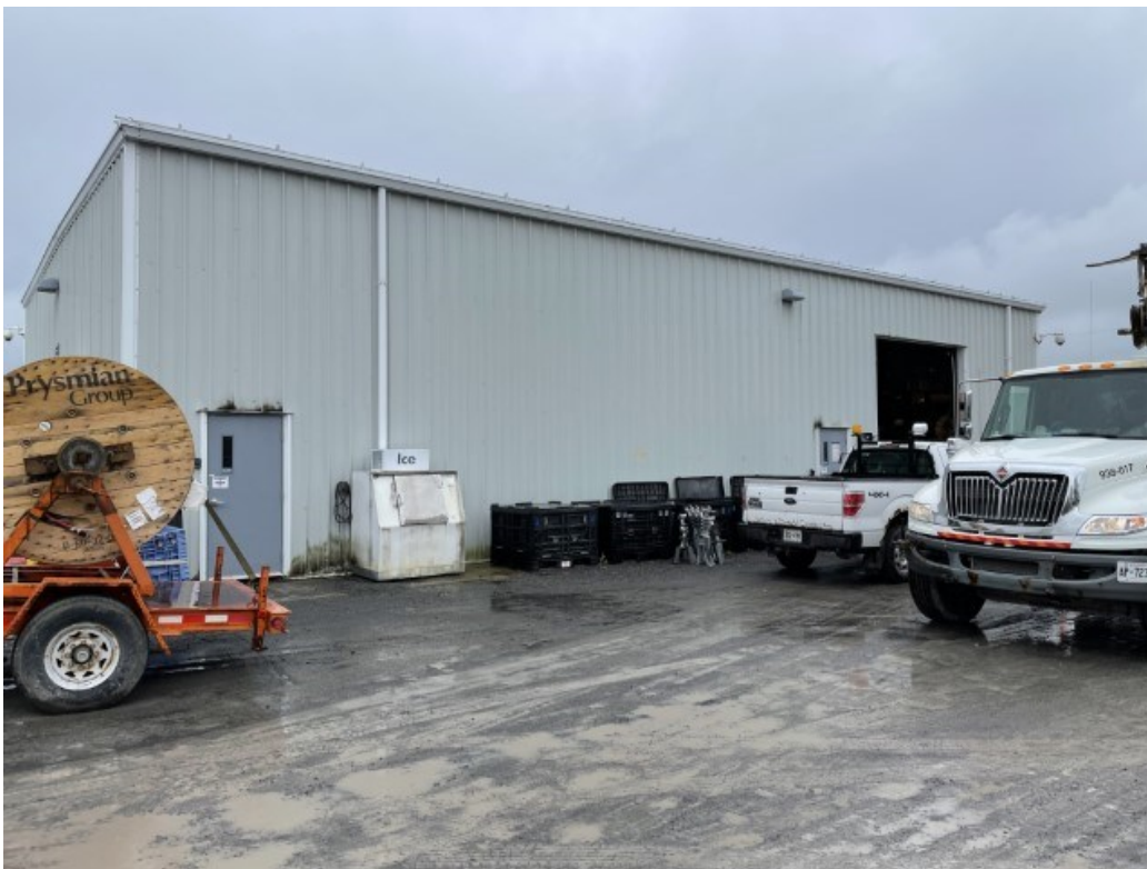
Photo 8: Warehouse building located in centre of Site, facing south
