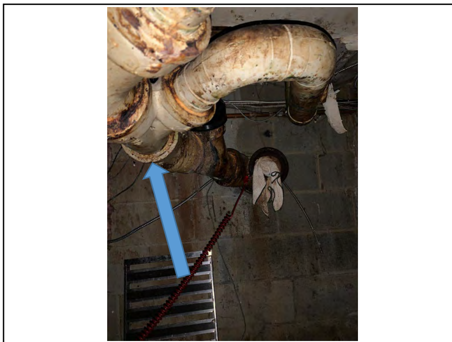
Photograph 19: View of cast iron drain along the south wall of the basement and suspected asbestos-containing oakum joint packing.
