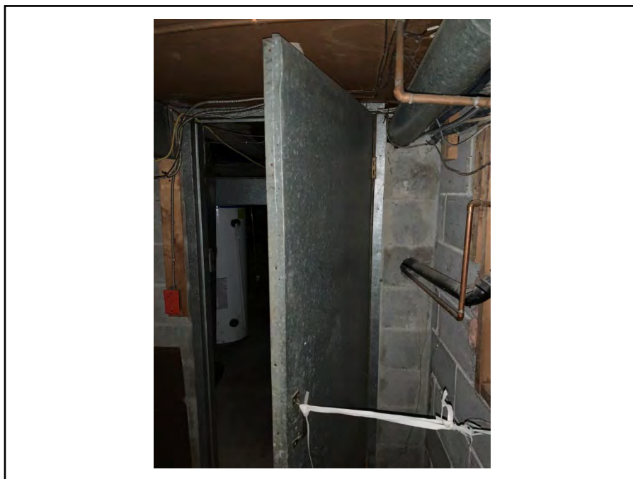
Photograph 15: View of fire resistant door in the basement furnace room with a suspected asbestos-containing interior liner.
