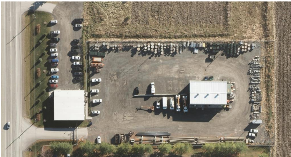
Figure 2 – Aerial View of Phase 1 HONI OC
