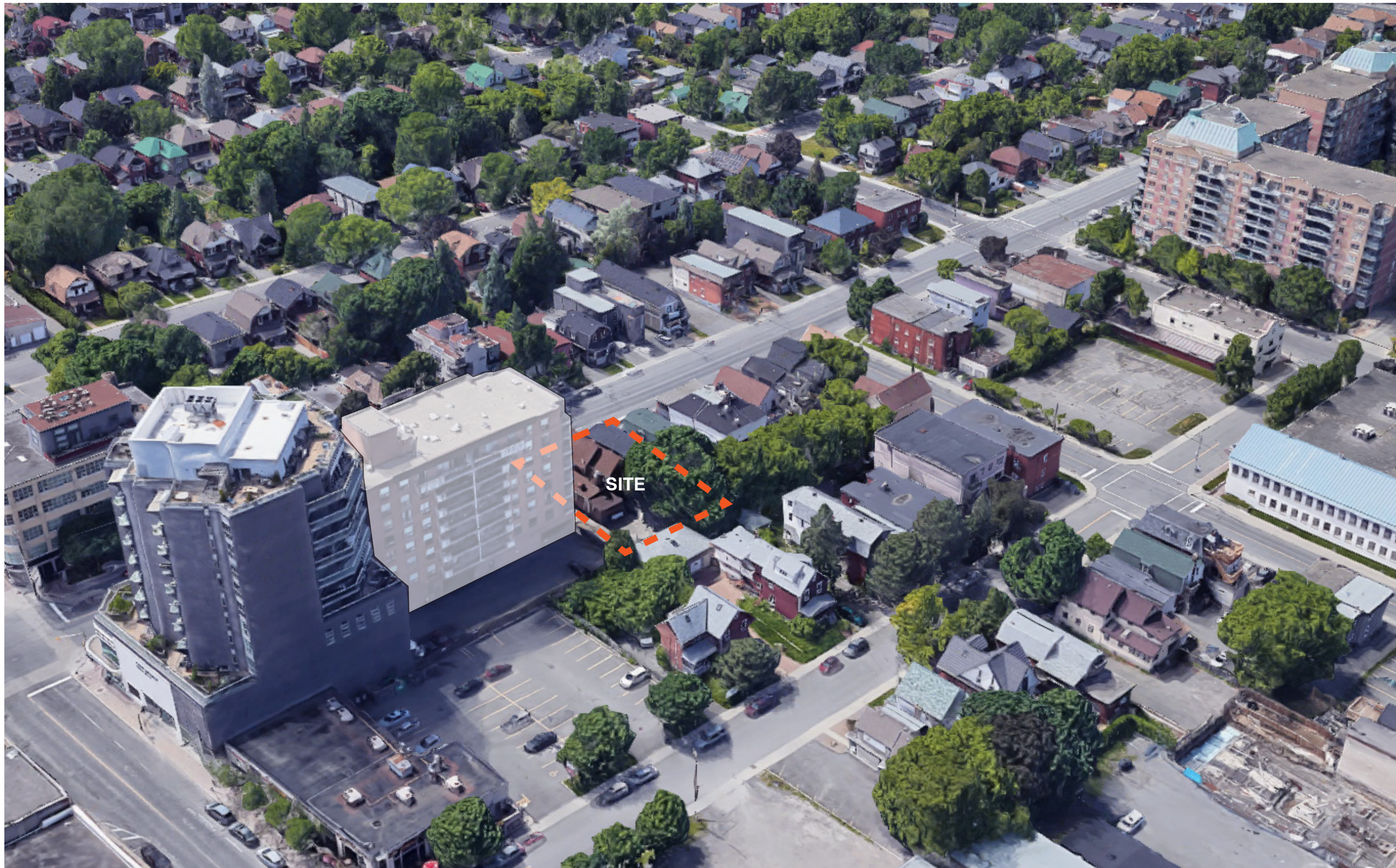
.9 AERIAL VIEW FROM NORTH EAST
