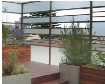
Image 4 – Example of a Porous Parapet around a Terrace
