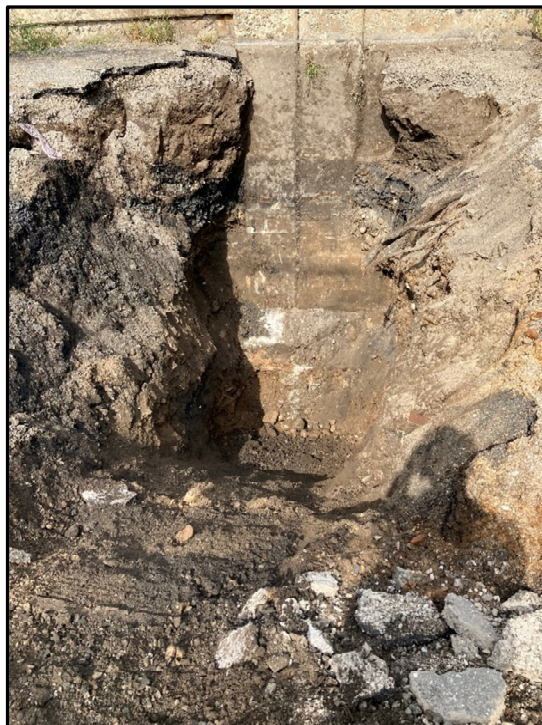
Photo 2: Photograph of the abutment footing in test pit TP 2-21.
