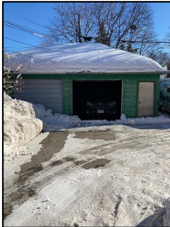
Photograph 2: View of private garage at the rear of 439 Churchill Avenue North.
