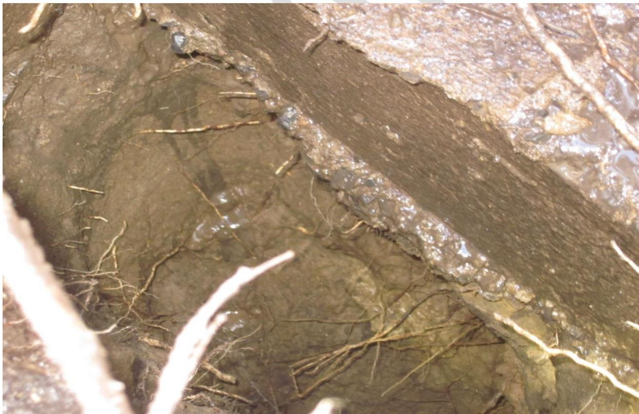
Picture 1. Typical size and number of roots encountered below concrete wall located at 667 Bank Street
