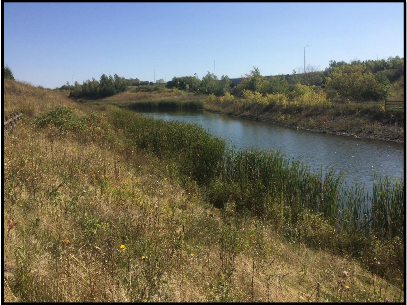
Figure 10: Steep slope and extensive disturbances associated with the construction of a stormwater management pond at the south edge of the study area. (PA1144-D37)
