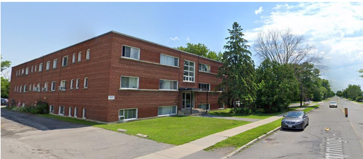
Photograph 2: Looking south along east side with 641 Cummings Avenue in the foreground.
