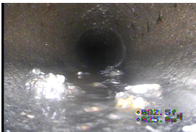
Figure#17: A view to the 10 % Debris ragging and sediment at 25.0 meters from the top of HALLWAY FLOOR CO.
