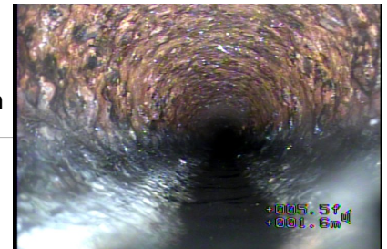
Figure#6: A view to the Pipe wall falling apart due to surface wear large at 8.2 meters from the top of the floor CO.
