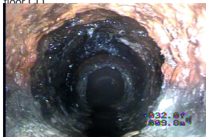
Figure#11: A view to the 150mm 12 o'clock connection at 16.4 meters from the top HALLWAY FLOOR CO.
