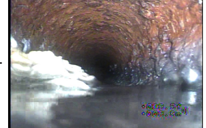
Figure#10: A view to the 50mm 12 o'clock connection at 11.8 meters from the top HALLWAY FLOOR CO.
