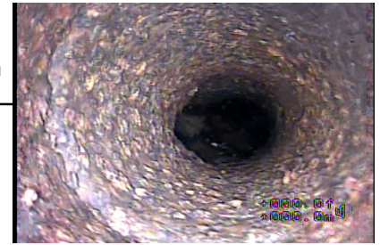
Figure#4: A view to the Surface Wear Large due to corrosion and grease at 1.6 meters from the top of the floor CO.
