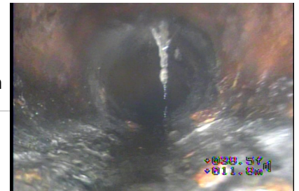
Figure#12: A view to the 100mm 12 o'clock connection at 19.4 meters from the top HALLWAY FLOOR CO.
