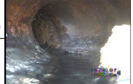
Figure#16: A view to the material change to Asbestos cement at 24.8 meters from the top of HALLWAY
