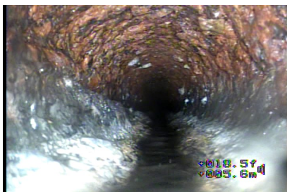
Figure#5: A view to the Roughness in the pipe walls and grease at 5.6 meters from the top of HALLWAY FLOOR CO.
