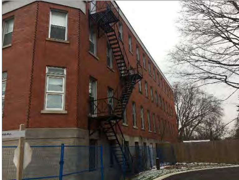
Photo 3 – Site Building (east elevation).
