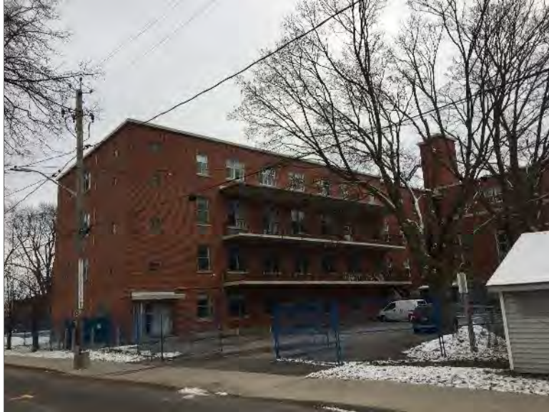
Photo 1 – Site Building (north elevation).
