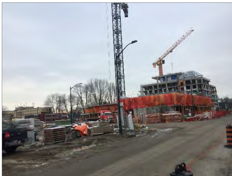
Photo 6 – Properties located south of the Phase One Property.
