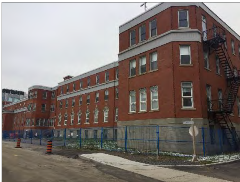
Photo 2 – Site Building (south elevation).
