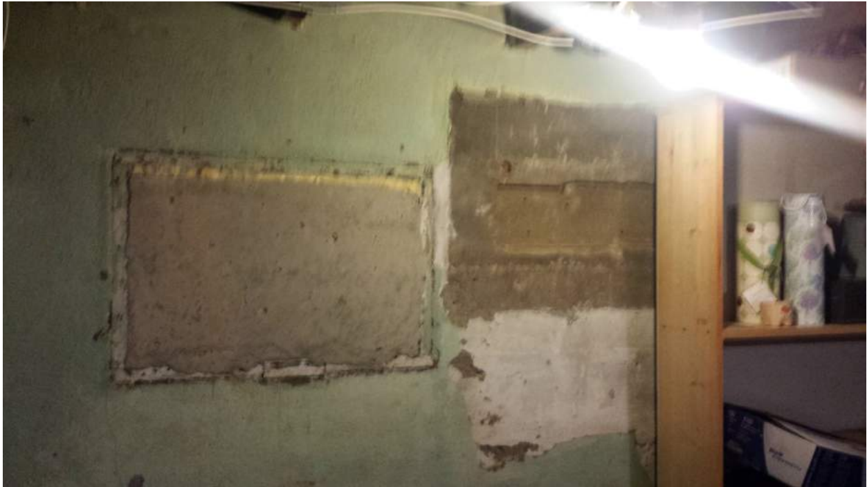
Photograph 7: The basement of 402 Roosevelt Avenue; former window or possibly a former coal chute.
