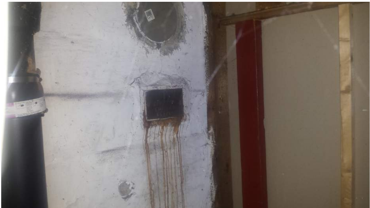
Photograph 8: Chimney cleanout at basement of 398 Roosevelt Avenue.
