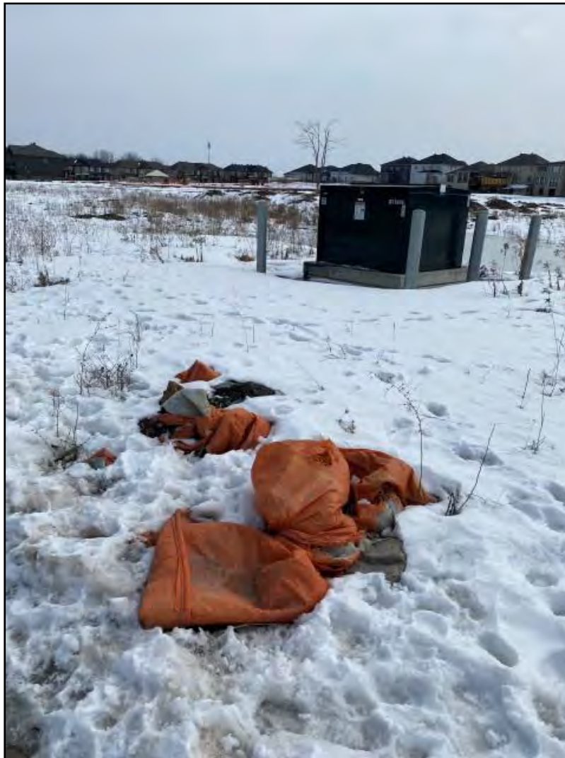
Photograph 10: Looking east at a transformer and construction debris on the west corner of the subject property.
