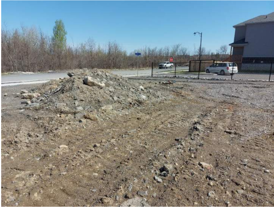
Photograph 3: Additional onsite fill piles
