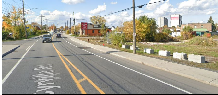
View 1: Looking Northwest @Cyrville Road
