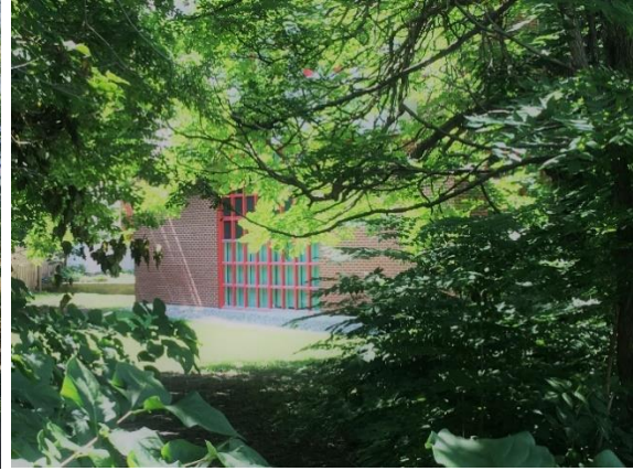
South facade Photo: City of Ottawa, August 2020
