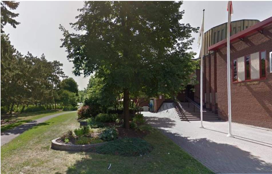
Looking south from Lewis Street. A multi-use pathway runs alongside the building. The CNA Dutch Tulip Celebration Garden is in the foreground. Photo: Google Street View - Jul 2018.
