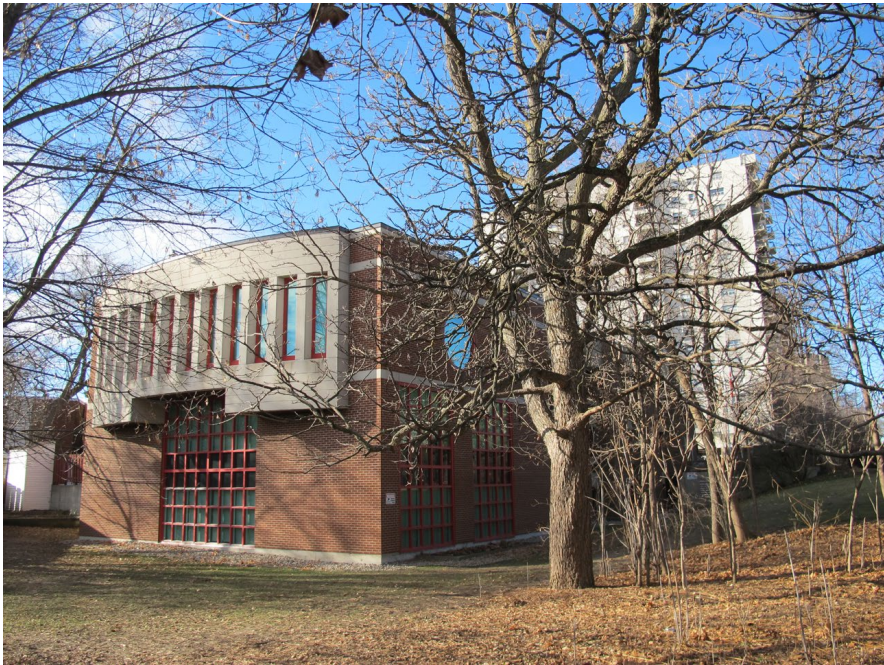
View NW of 1987 addition
