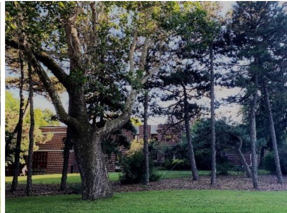
East façade, looking west Photo: City of Ottawa, August 2020
