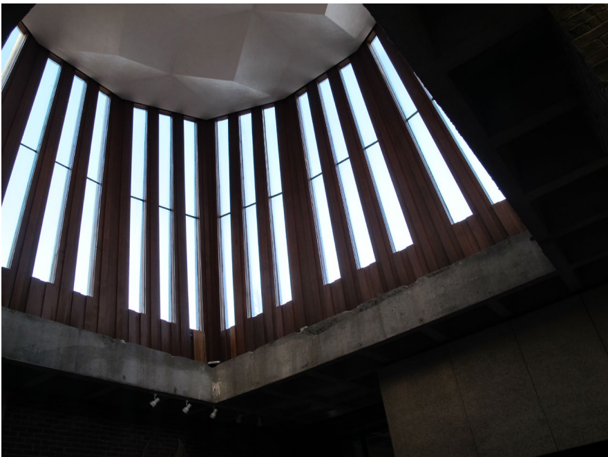
Underside of lantern
