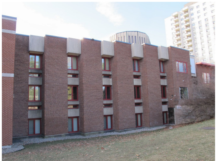
Front elevation south portion (1966 building)
