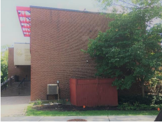
North façade Photo: City of Ottawa, August 2020
