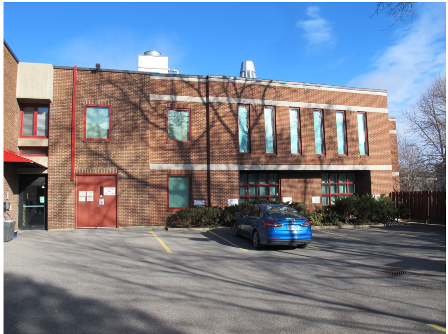
Rear elevation (1987 addition)
