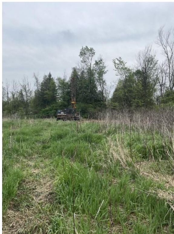
Photo B: Geotech
