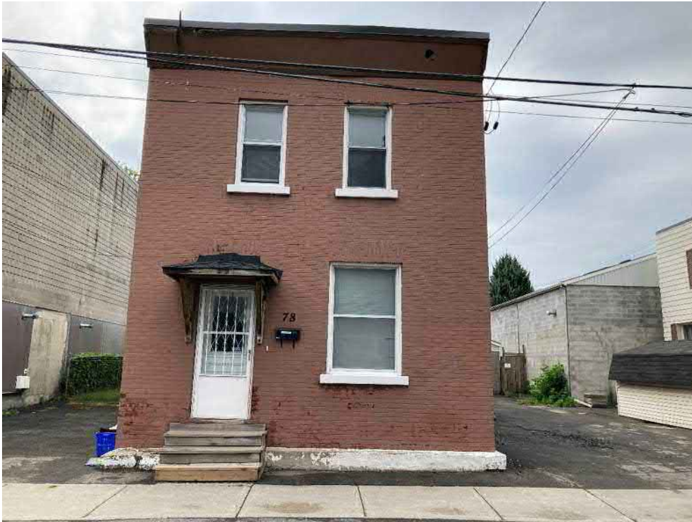
Photo 1: View of the main entrance to the building, looking west.
