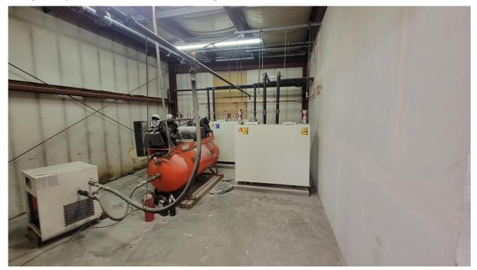
Photo 2: Facing Northeast, second floor northeast corner of the Site building. Three 2200L Active ASTs containg engine oil along with a compressor present.
