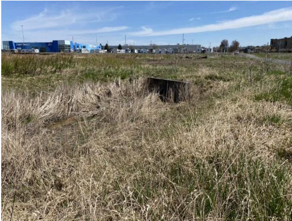
Photo 3: Stormwater culvert entering ditch
