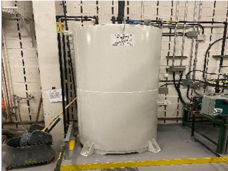
Photo 8 – 1,663-L double-walled steel AST containing diesel located in the northwest portion of Site Building B (PCA/APEC).
