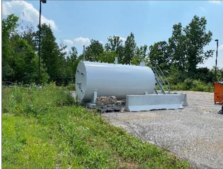
Photo 7 – 24,974-L steel AST, reportedly empty and not in use, located exterior to the southwest elevation of Site Building B (PCA/APEC).
