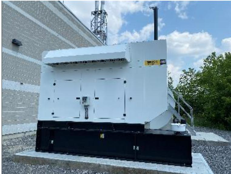
Photo 6 – 1,544-L belly tank steel AST, associated with an emergency generator, located exterior to the southwest elevation of Site Building B (PCA/APEC).
