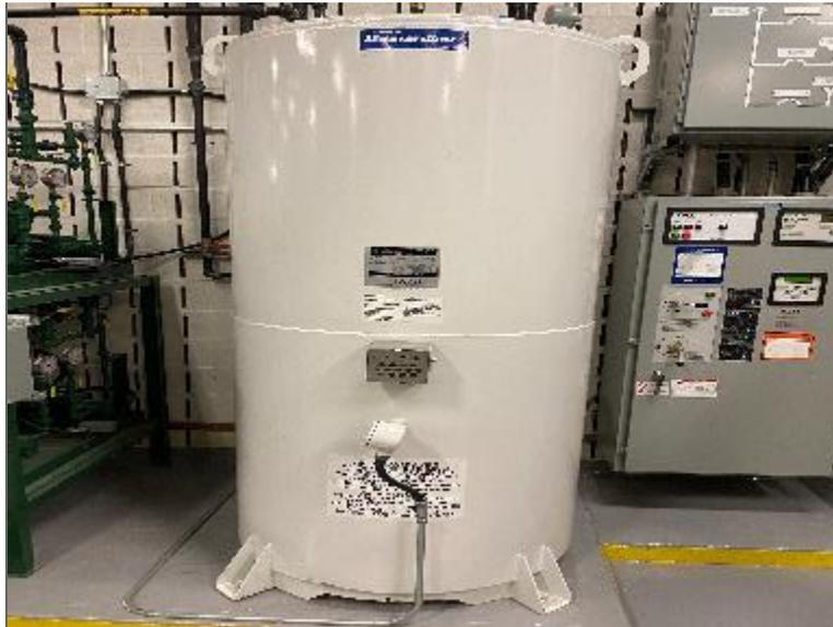
Photo 10 – 1,663-L double-walled steel AST containing diesel located in the southeast portion of Site Building B (PCA/APEC).
