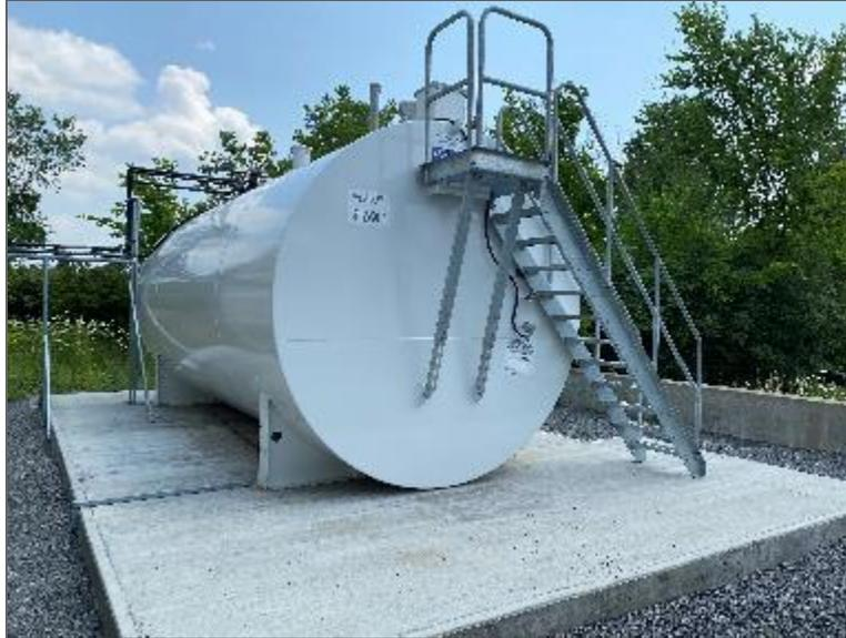
Photo 5 – 45,698-L double-walled steel AST located exterior to the southwest elevation of Site Building B (PCA/APEC).
