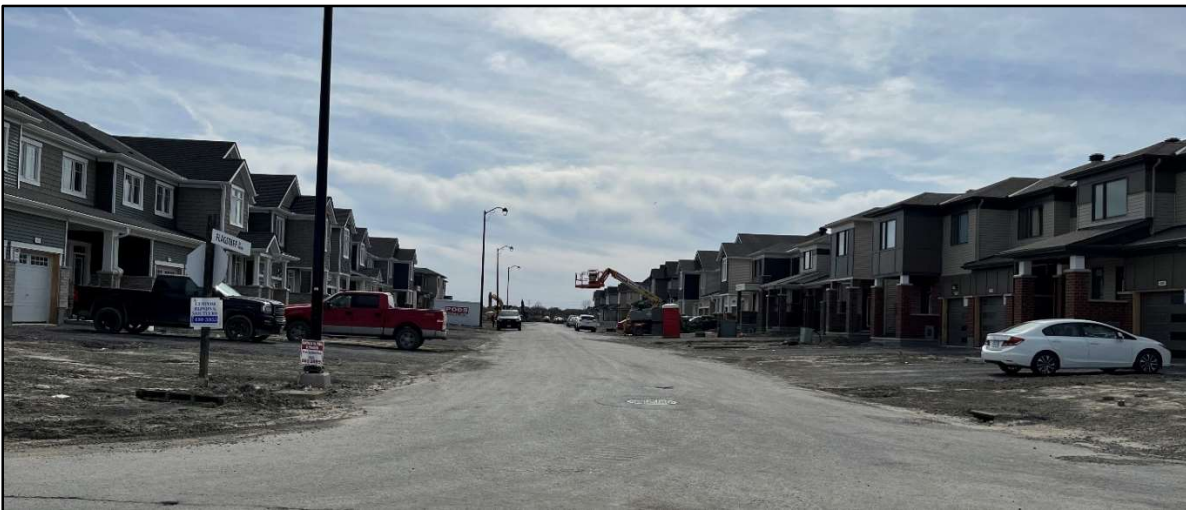
Exhibit H: Photograph facing west on Flagstaff Drive with recently constructed townhouses by Mattamy
