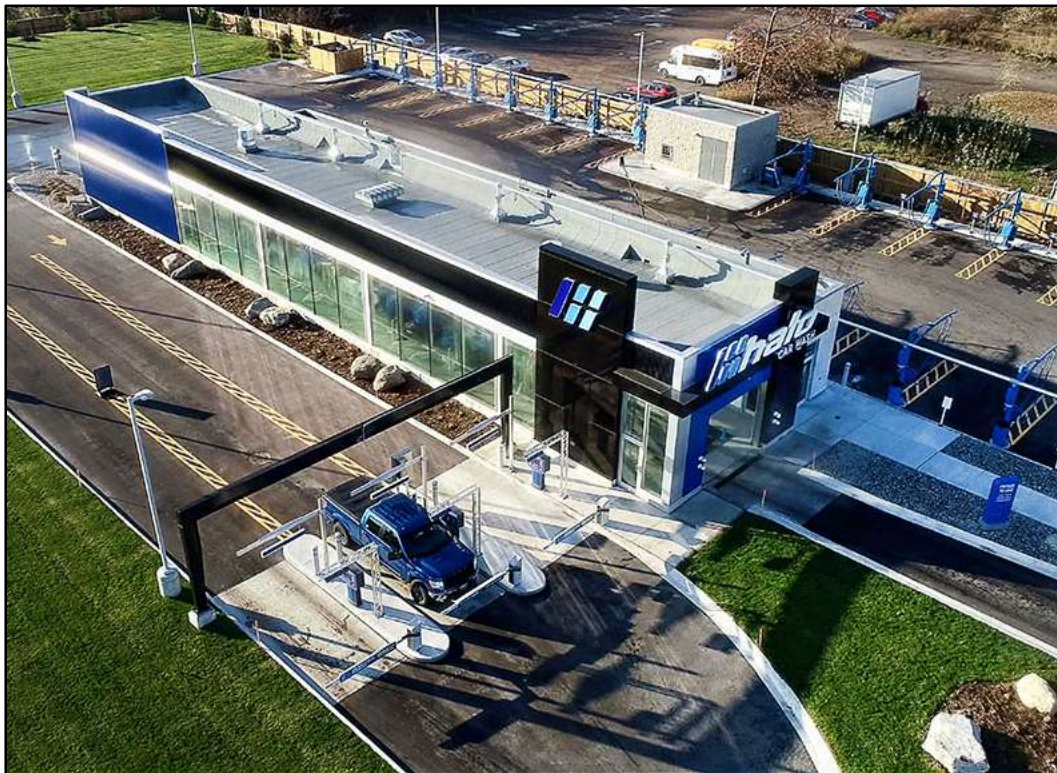
Exhibit K: Typical Halo Car Wash layout with three queuing lanes and entrance arch (foreground), wash tunnel and vacuum stalls (background) (Pictured: 3604 Innes Road, Ottawa)
