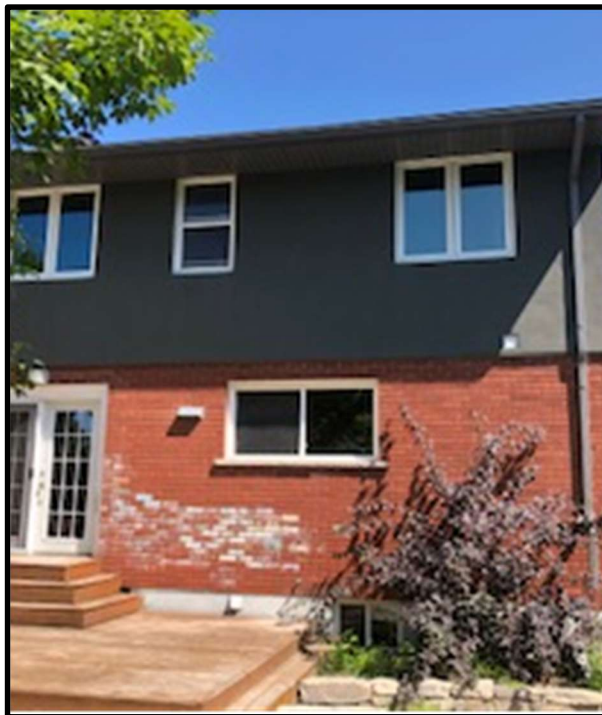
Photograph 2: Rear view of subject building looking east.
