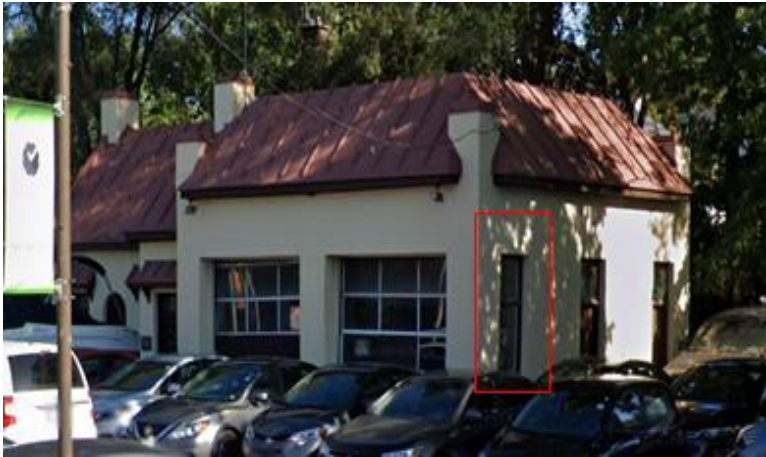
Figure 31: View showing the side elevation of the Service Station with three windows. The proposed midrise building has been set back and allows one of the side windows to be interpreted. Source: City of Ottawa.
