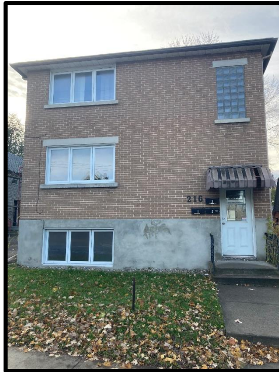
Photograph 1: View of the front of the residential triplex building addressed 216 McArthur Avenue, facing south.
