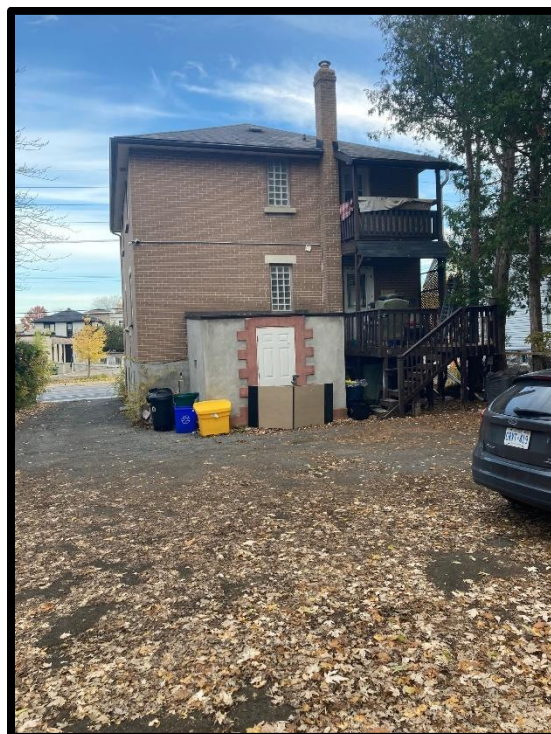
Photograph 2: View of the back of the residential triplex building addressed 216 McArthur Avenue, facing north.
