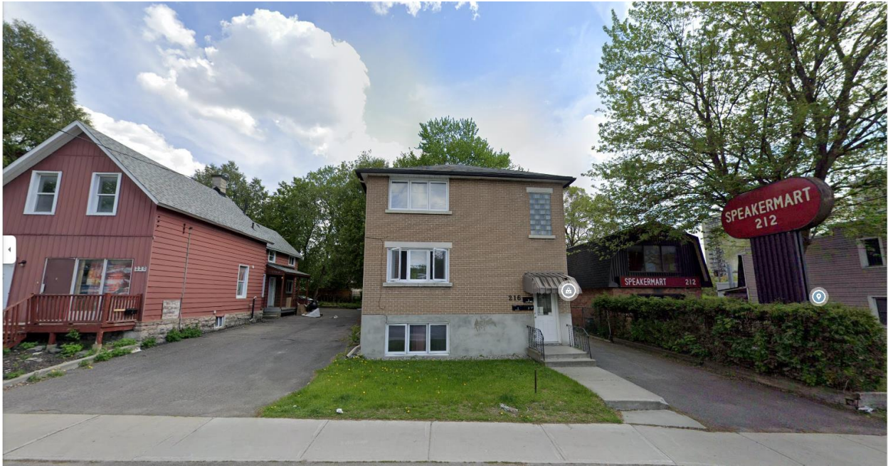
Figure 1: 216 McArthur Ave – Existing Building
