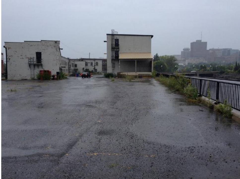
Photograph 15: Paved ground of the Phase One Property on Albert Island, facing east (August 12, 2014).
