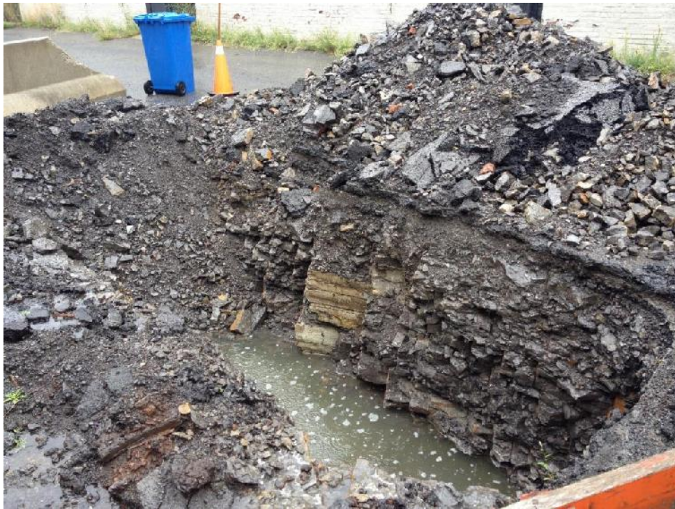
Photograph 16: Fill and shallow bedrock observed in an excavation on Albert Island (August 12, 2014).
