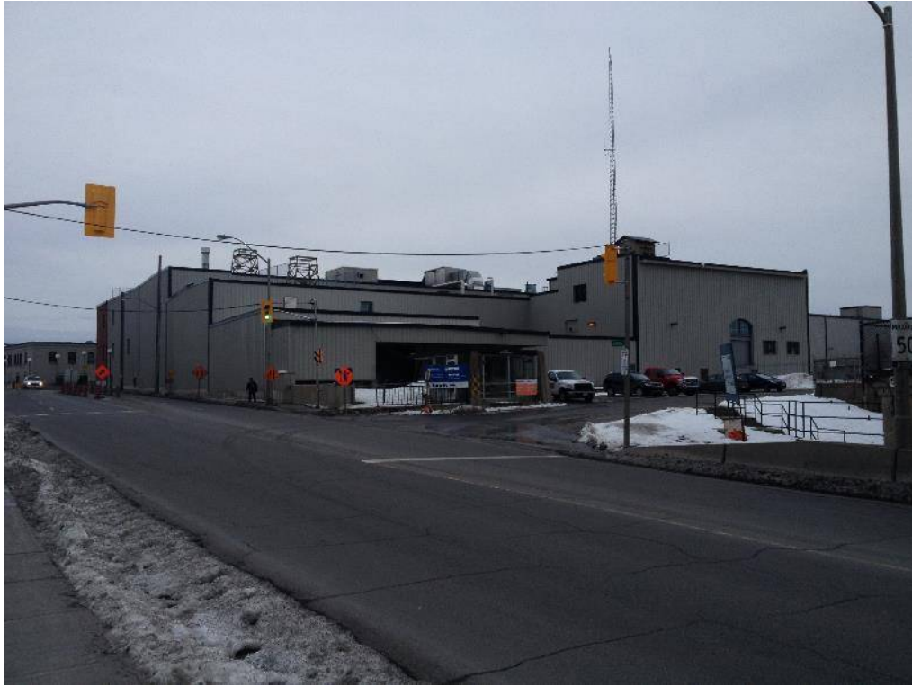
Photograph 1: View of north side of former paper mill, facing south (April 7, 2014)
