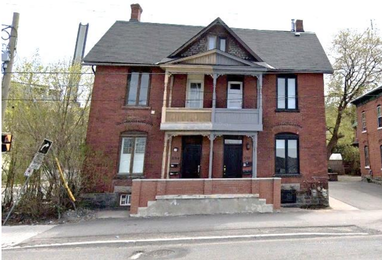
Figure 19: 684-686 Albert Street. Source: Google streetview, image May 2019.
