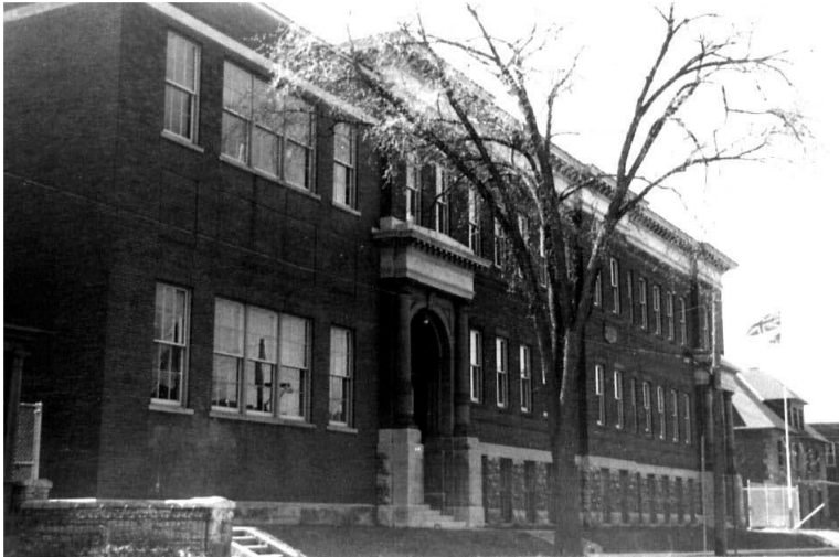
Figure 10: Wellington Street School, built after the fire of 1910, and located on the 665 Albert Street on the site of what had been the Charles Pinhey estate. Photo taken in 1962. Source: City of Ottawa Archives, CAO CA 21047, reproduced in Past Recovery Archaeological Services, Stage 1 Archaeological Assessment of LeBreton South, Parts Lots 39 & 40, Concession A, Ottawa Front , 2012: Image 14.
