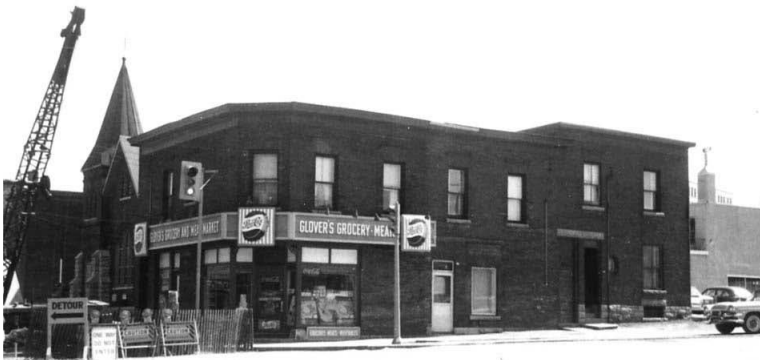
Figure 12: Buildings located on the east side of Booth Street between Albert and Wellington street, on the site what is now 665 Albert Street, in 1962. Source: City of Ottawa Archives, CAO CA 21054, reproduced in Past Recovery Archaeological Services, Stage 1 Archaeological Assessment of LeBreton South, Parts Lots 39 & 40, Concession A, Ottawa Front , 2012: Image 17.
