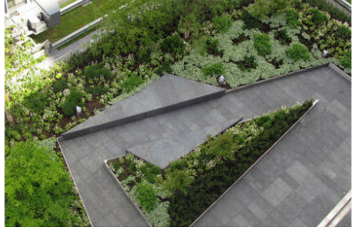
Figure 5.13 : Example of a green infrastructure to protect the building from direct solar heat and reduce urban heat effect.
