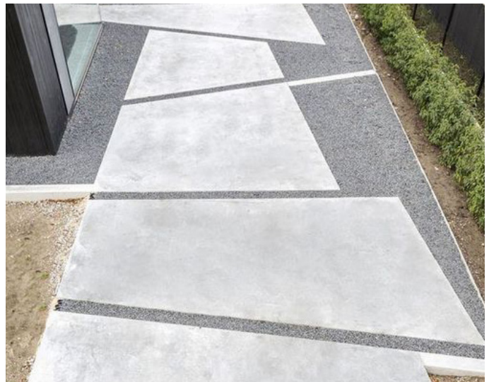
Figure 5.17 : Example of pedestrian walkway with permeable surfaces and reflective materials to reduce heat island effect.
