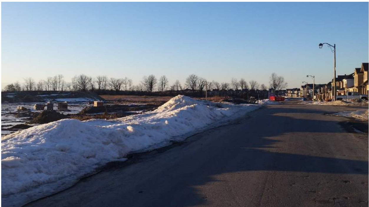
Photograph 8: North part of the subject site, looking north from Alex Polowin Avenue.
