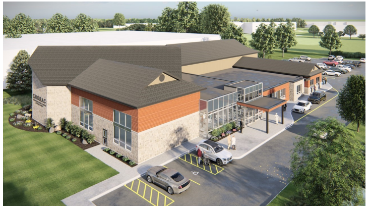
ABOVE RIGHT: The majority of parking is located at the rear of the site and will be screened from the public street by the proposed church. Barrier free parking has been located at the front of the site with direct access via an accessible sidewalk to barrier free building entrances.
