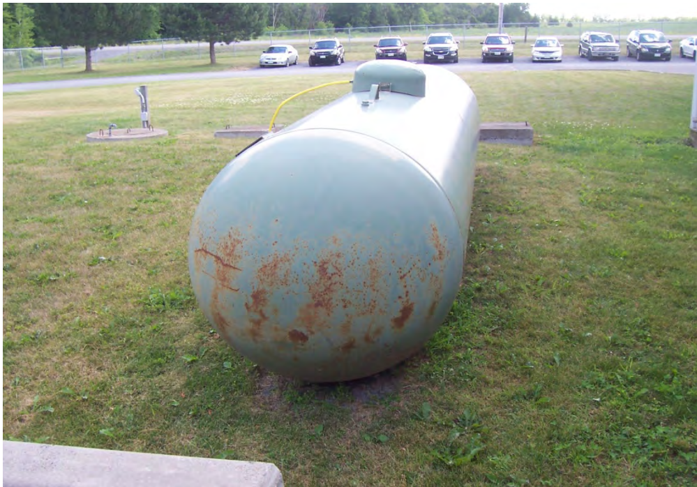
Photograph 9: Propane tank located north of the maintenance garage with the septic tank and septic field in the background.
