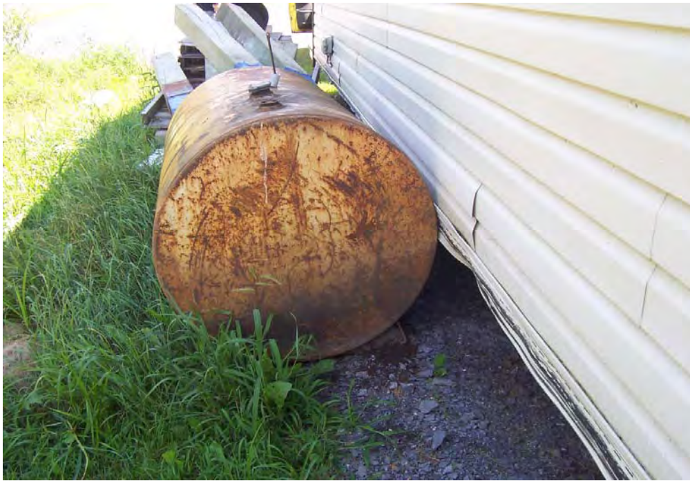
Photograph 5: Former waste oil tank located along the north wall of the tire storage trailer.
