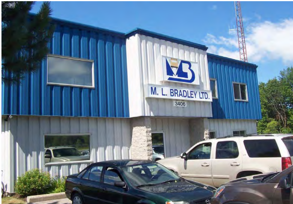
Photograph 1: Front entrance to the M. L. Bradley Site at 3406 Frank Kenny Road in Ottawa, Ontario.
