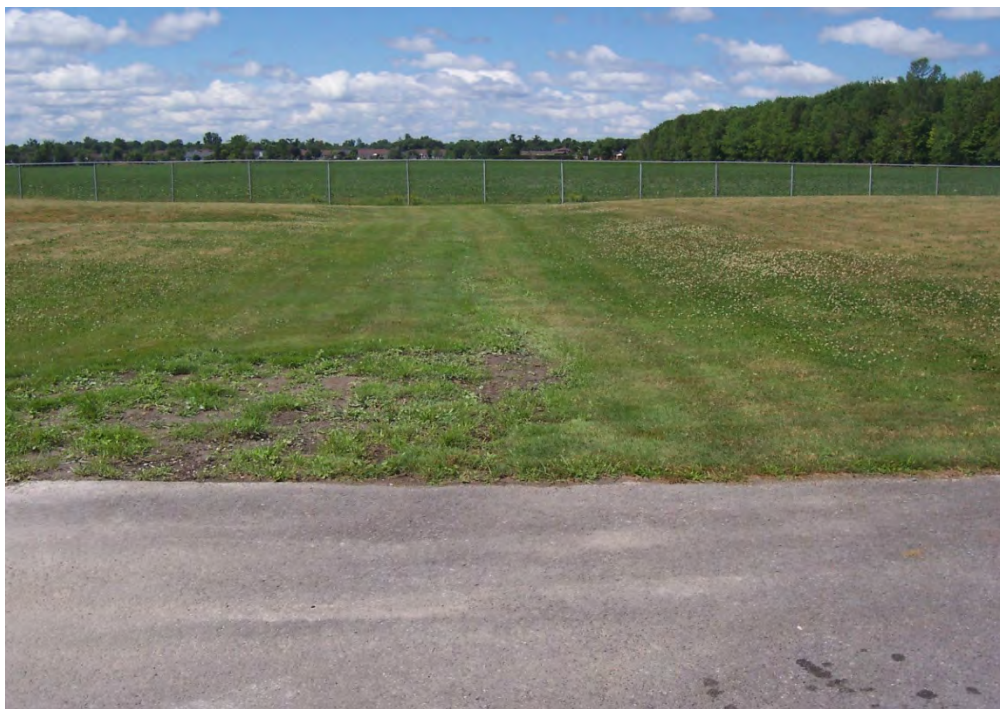
Photograph 12: Swale that allows surface water to drain to the west off-site.
