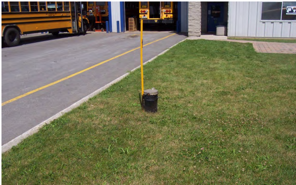
Photograph 10: One of two ground-source wells located at M. L. Bradley.
