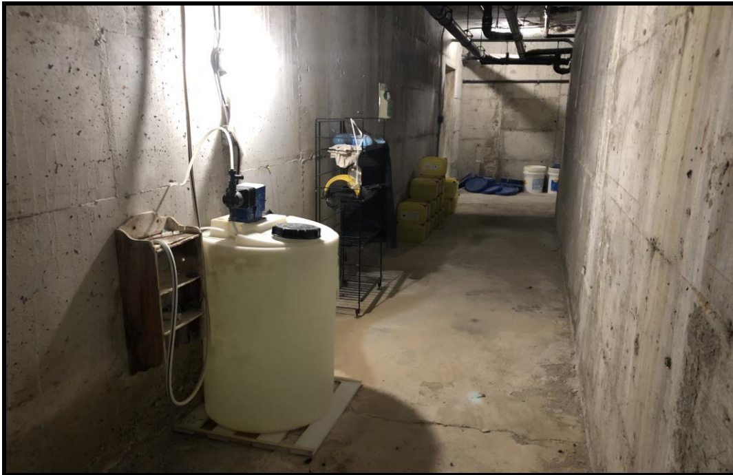
Photograph 6: View of a chlorine storage drum and several small chlorine storage containers, located in the basement of the recreational amenity building.
