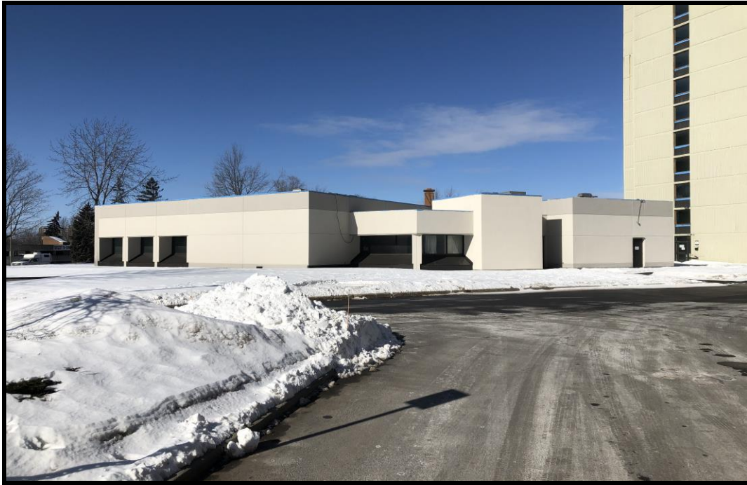
Photograph 1: View of the southern portion of the subject site, facing north.
