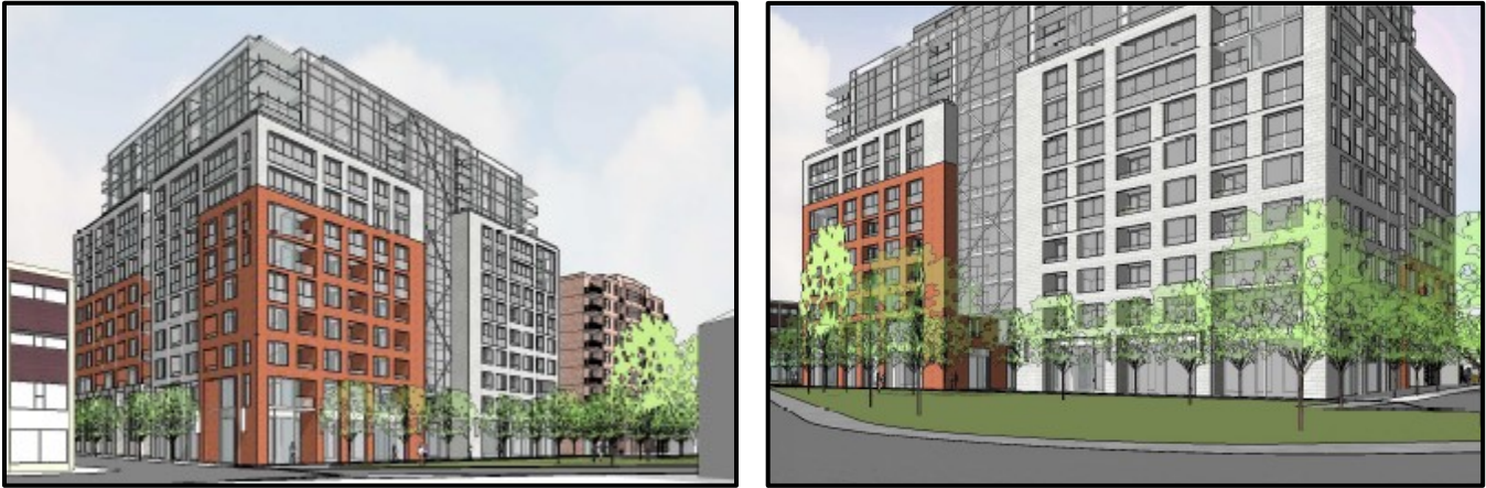
Figure 12: Wellington Street West frontage
