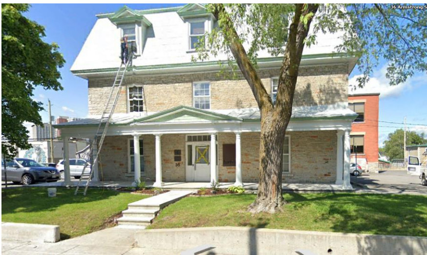
Figure 6: View the Armstrong House designated under Part IV of the OHA. Note the mansard roof, a feature that dates to the conversion of the building to a convent. Banfield Marketing Agency presently occupy it. Source: Google Earth
