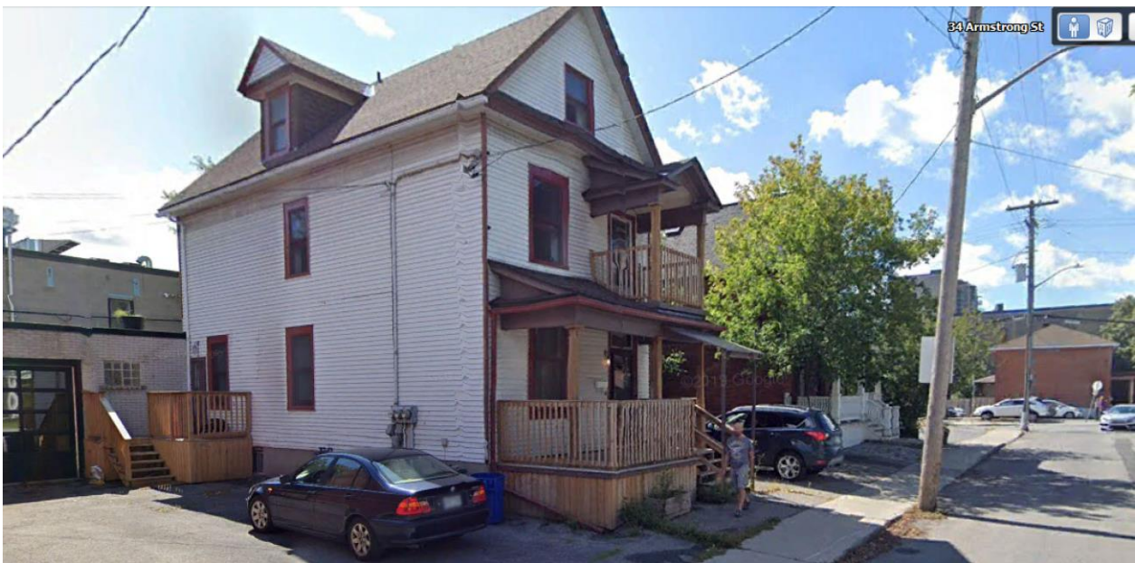
Figure 9: View of 36 Armstrong with 40 Armstrong to the right. Source: Google Earth
