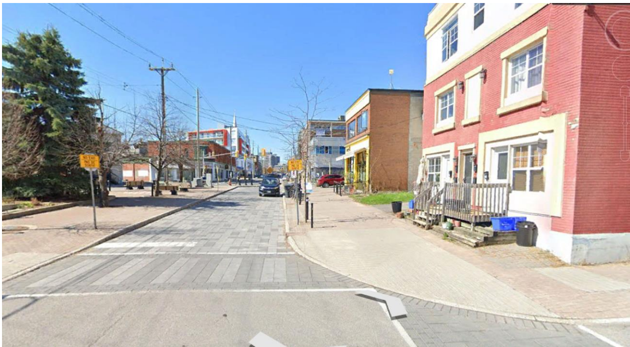
Figure 3: Street view looking west on Wellington Street from Hilda Street, 967 Wellington to the right, is part of the proposed development lands and the building is planned for demolition. Note the irregular street setbacks, brick cladding and flat roofs. Source: Google Earth
