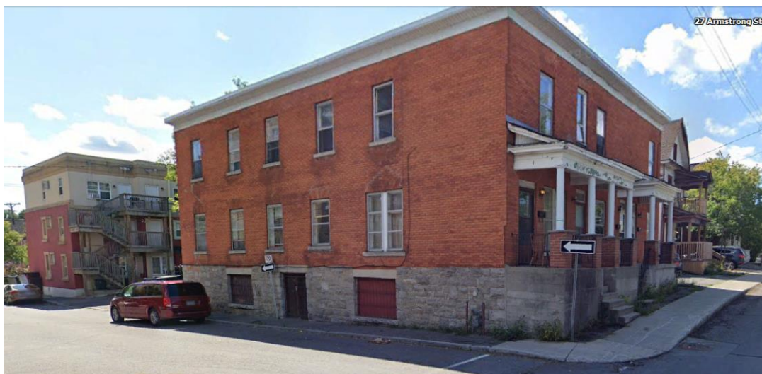
Figure 7: View of the row house at 26 Armstrong (right) and 967 Wellington (left) with no accessible frontage on Hilda Street. The building is typical of the area’s character– two and three storey brick clad building, masonry foundation with flat roofs set on the property line. Both buildings on this block of Hilda Street are slated for demolition. Source: Google
