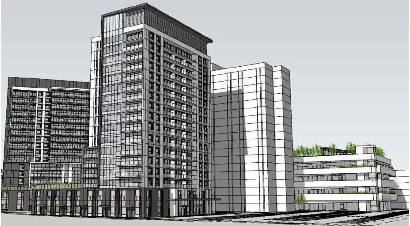
Figure 12 Building C, surface parking area, and Parking Garage from St. Laurent (Existing high-rise in background).
