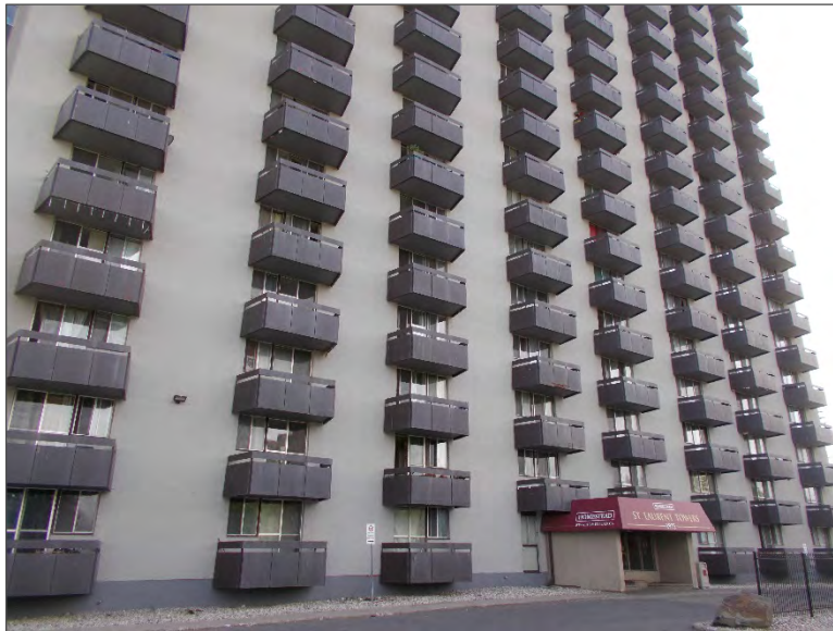
Photo 4 – Site Building B (north elevation).
