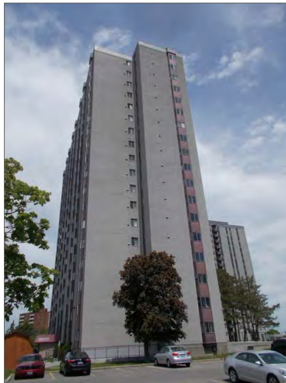
Photo 2 – Site Building A (south elevation).
