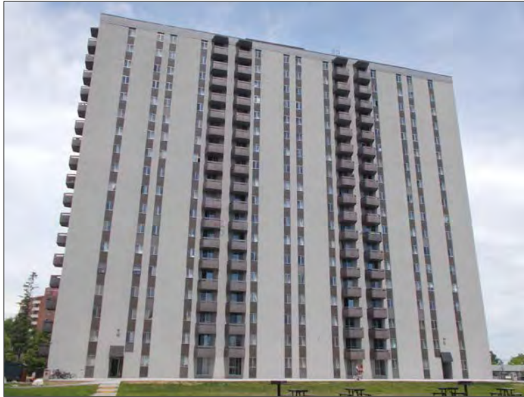
Photo 3 – Site Building B (south elevation).
