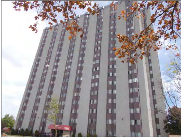
Photo 1 – Site Building A (west elevation).
