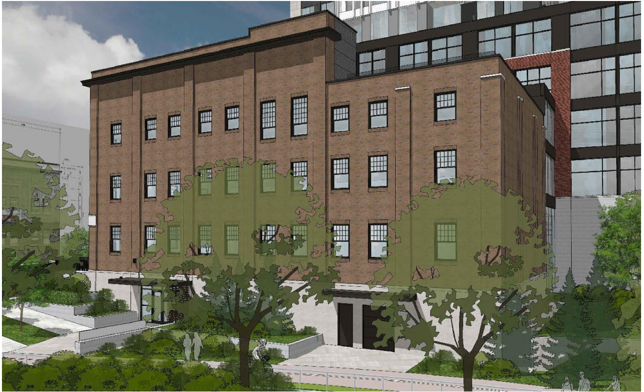
Figure 19: Rendered perspective view of the east elevation of the Standard Bread Building with the multi-use path system in the foreground. The fenestration pattern provides reference to the original openings, a number of which have been bricked in and will be opened up. The documented fenestration pattern will be retained. Source: Hobin Architecture 2021.
