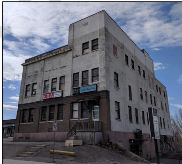
Photo 1: 951 Gladstone Avenue, south and east elevations [JCAL 2018].
