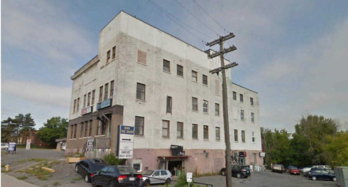
Figure 3: View looking west along Gladstone to the development site. Note the fenestration pattern on the east elevation (left) which characterizes its light industrial use with doors occurring on the second and third-floor levels and the location of an internal hoist to move material between floor levels. Source: Google Earth.
