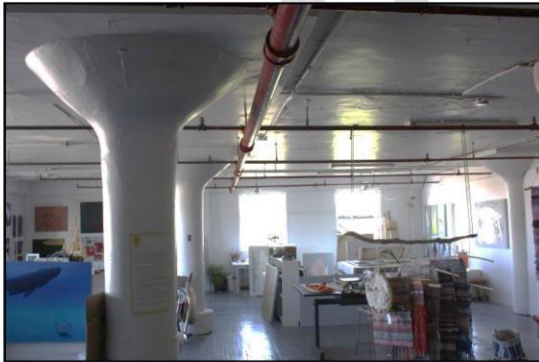
Photo 2: Typical columns inside the building [JCAL 2018].
