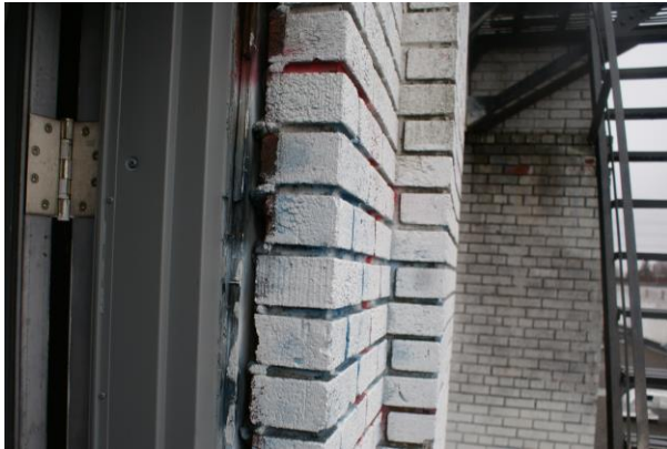
Figure 32: View of the exterior brickwork from a second-floor fire escape. Note the highly textured brick surfaces and recessed joint profile. Source: Commonwealth 2020.
