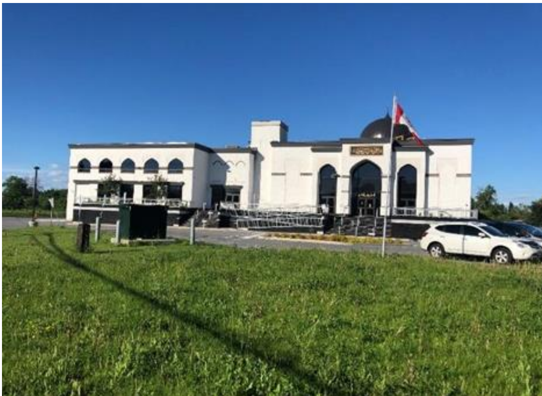
View to Jami Omar Mosque from existing vacant lot, 3990 Old Richmond Road (June, 2019)
