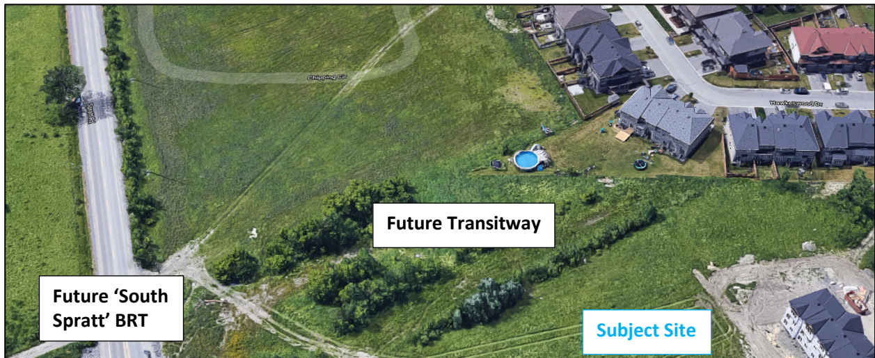
Figure 5: Looking south from above the Subject Site
