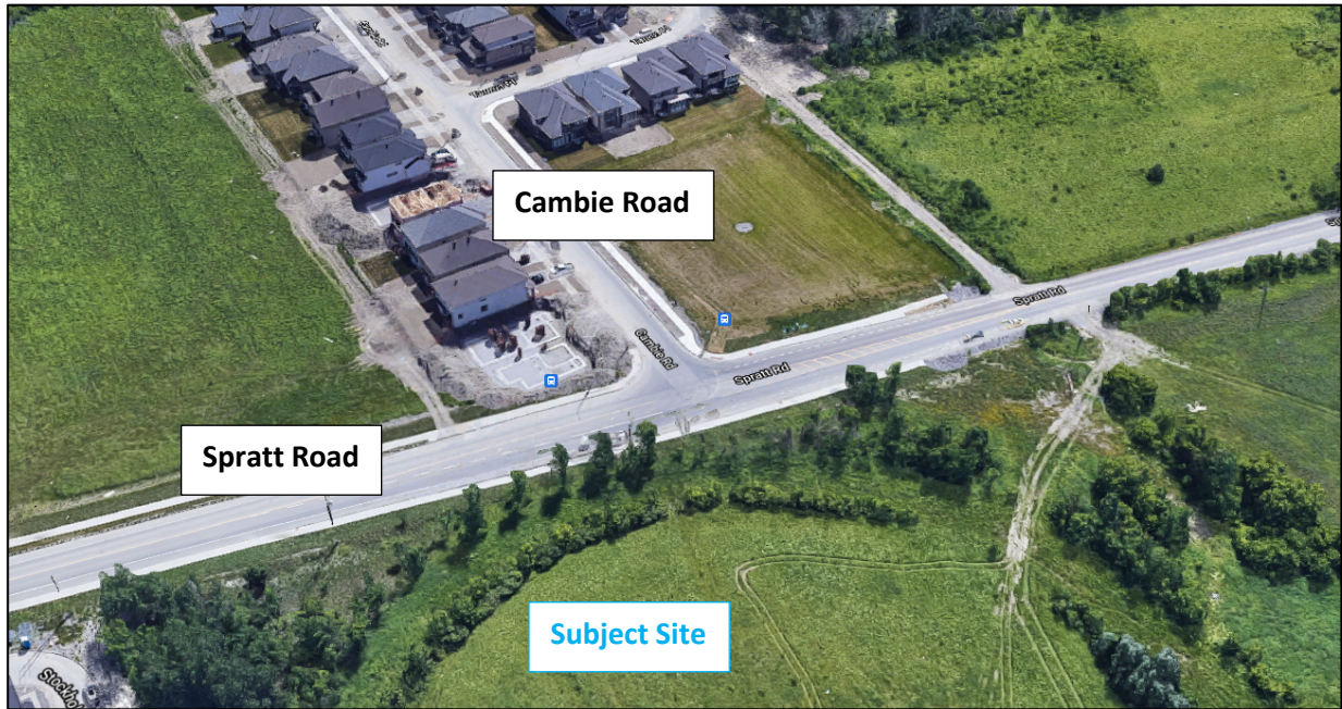
Figure 4: Looking east across Spratt Road from above the Subject Site
