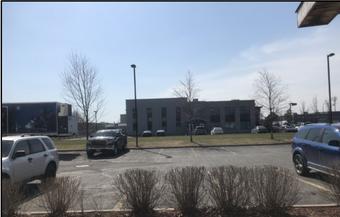
Photo 7: South-facing view of adjacent commercial buildings.
