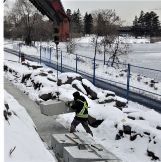
Blocks being set in place with a backhoe and chain.
