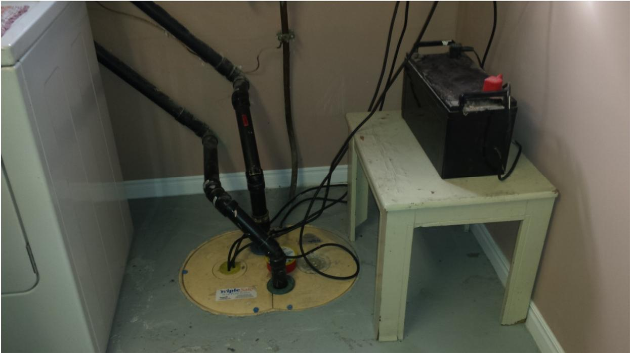
Photograph 3: Sump pit (with two submersible pumps) and backup battery in the basement of 3996 Innes Road.
