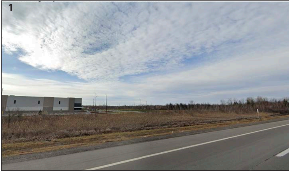
View southeast toward the site from the eastbound lane of Highway 417 - Amazon's distribution warehouse can be seen to the left (Fall)
