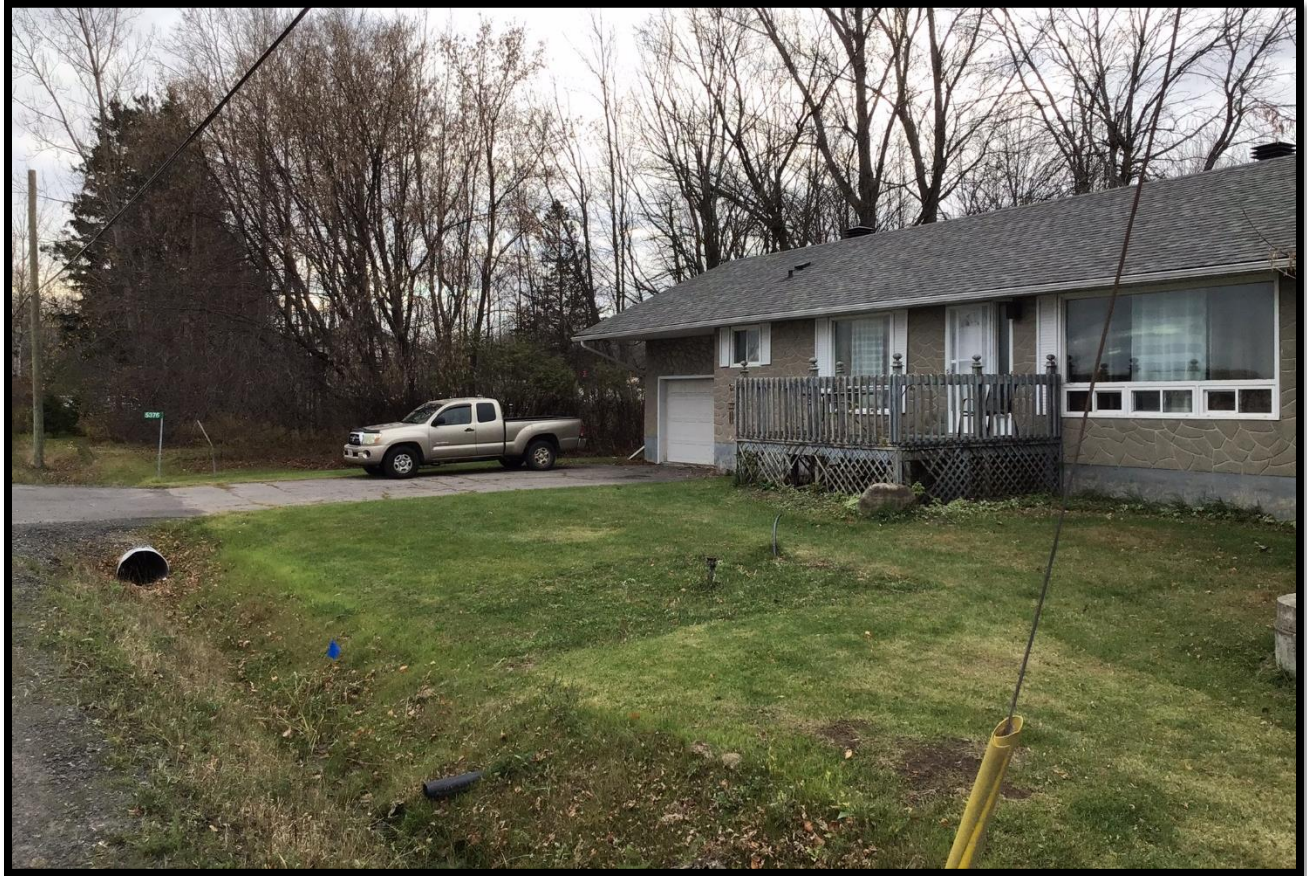
Figure 7: Residence and built-up property at 5376 Boundary Road. (PA1164-D46)
