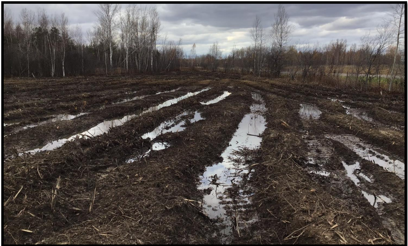
Figure 12: Extensive disturbances from recent grubbing. (PA1164-D08)
